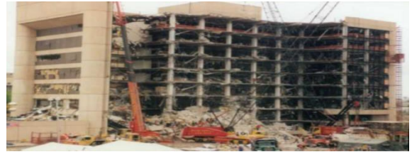
Fig.1. Progressive collapse in Alfred P Murrah
