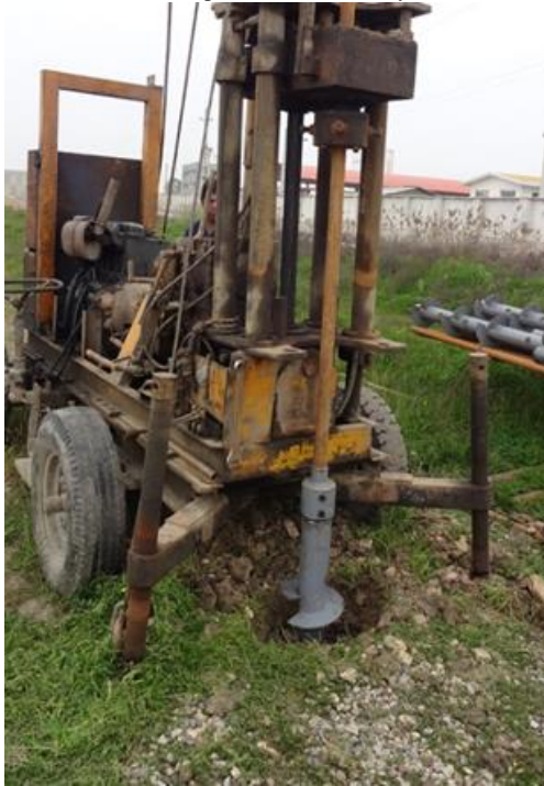
Figure 5. Helical pile installation equipment
